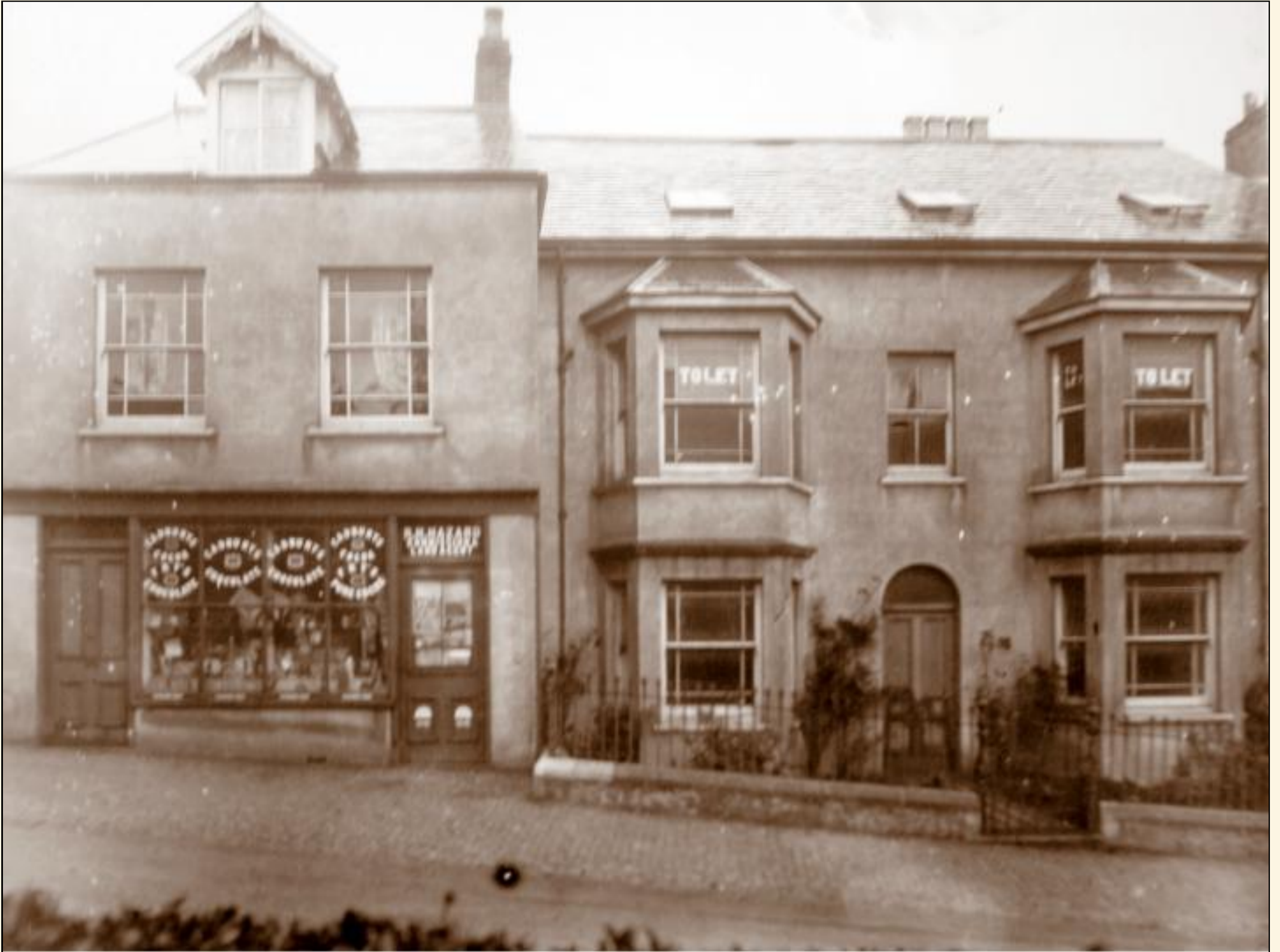
He subsequently rebuilt it as can be seen in this slide, but after another fire he gave up and the site next to Peria is still vacant today.
