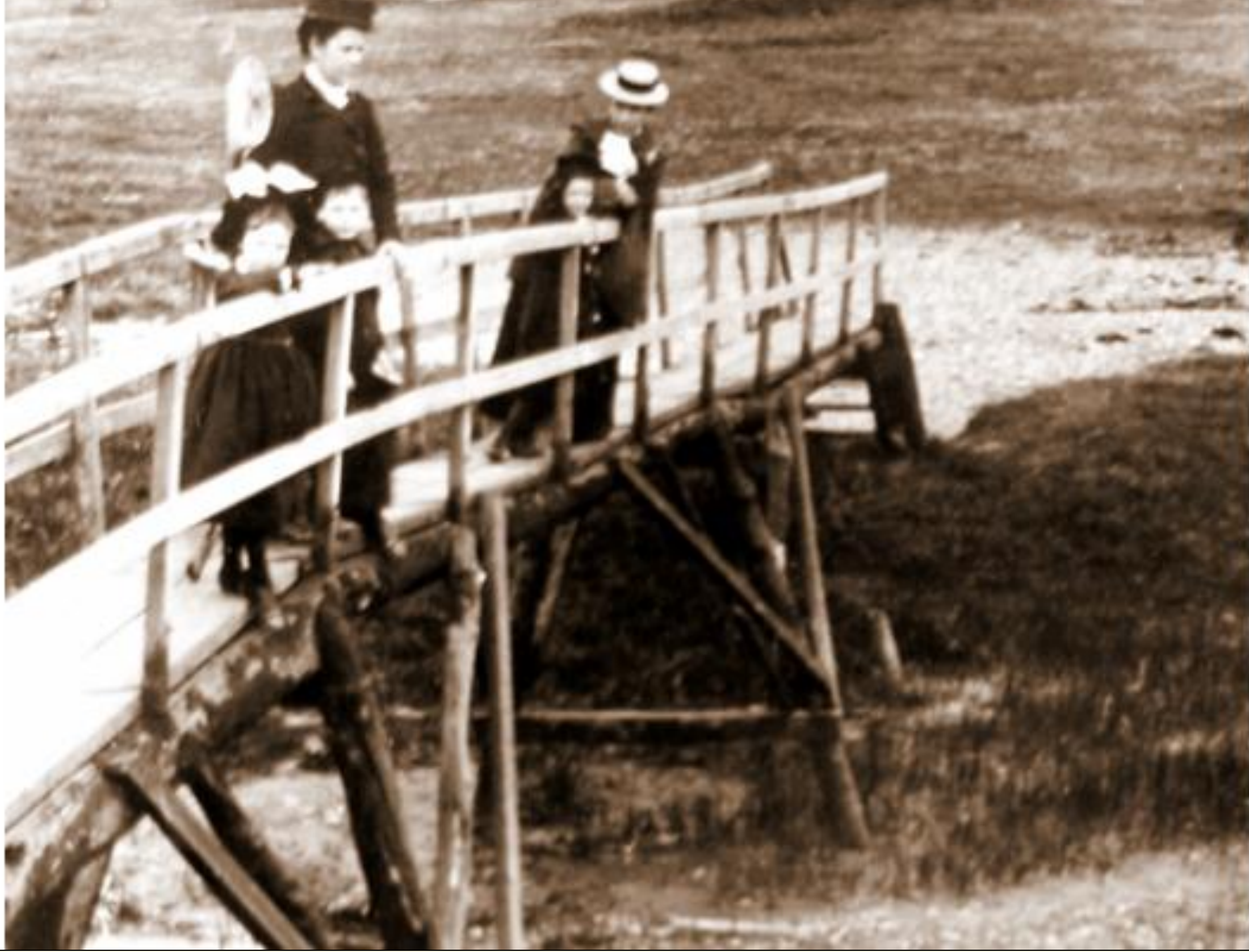
In 1897 Queen Victoria was commemorated by the construction of "The Jubilee Shelter". It had formerly been the building used to store the ammunition for the Volunteers but was adapted by adding a roof and balcony around it, as can be seen in this photograph of the timber bridge that went over to the island where it stood.
